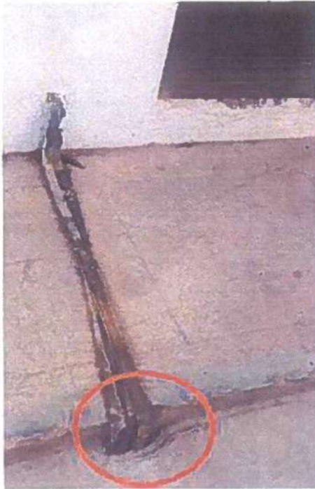
Earth pit NOT traceable, interconnections with Bolts not allowed, should be braised
