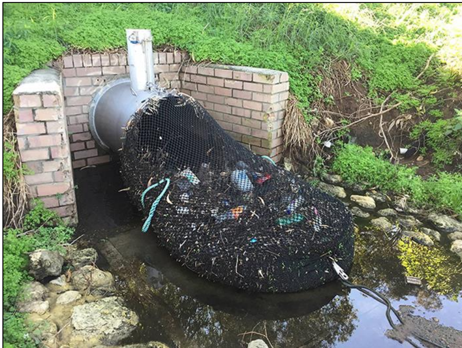
Fig 4.2: Solid waste collector fitted at the mouth of the sewage pipe
